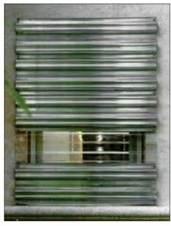
**TIP:** You can bring more light into the house by adding in some clear Lexan panels, which are shaped the same as the metal ones and install the same way (**left**).
