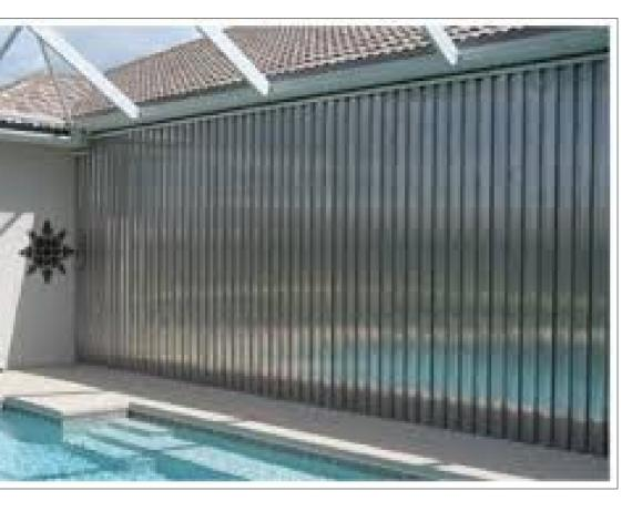
These heavy and sharp-edged metal panels are corrugated, and install overlapping each other, and so are very resistant to strong winds and debris.
